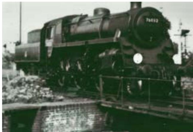
1911 saw the construction of two new sidings to facilitate the heavy excursion traffic in the summer. The platforms were also lengthened and the turntable was enlarged to cater for the larger engines needed to pull the excursion trains. This turntable is now buried under the current car park.
